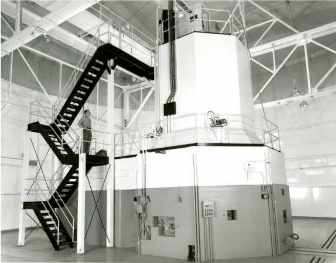
Figure 7. Inside Building 280 with the LPTR, shortly after construction, looking south, 1957.
