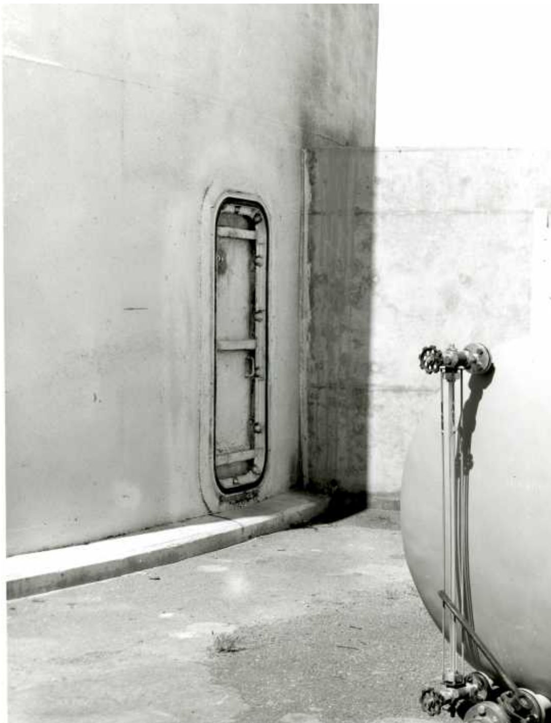
Figure 15. Escape air lock door at Building 280 at left, with connection to Building 281 at right, 1961. LLNL Archives.
